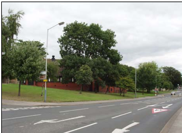
Open space surrounding Swanwick Memorial Hall
