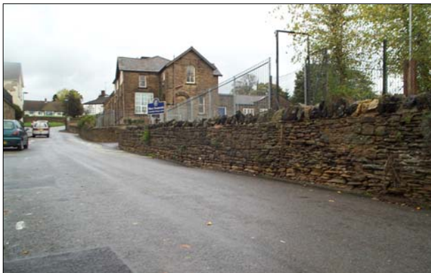
Stone wall along Church Street North
