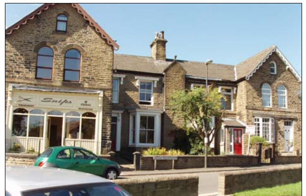
Nos. 1-7 (odd) Church Street North
