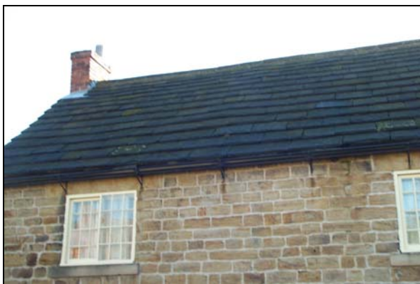
Traditional stone roof
