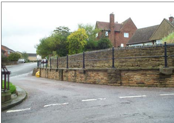
The raised pavement
