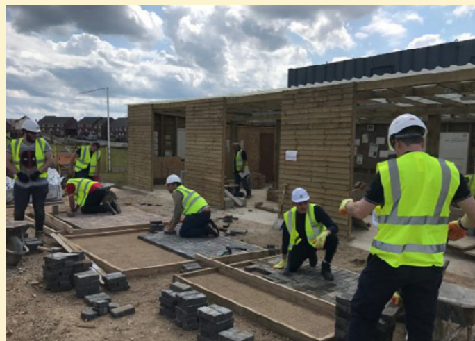
Scarborough Construction Village – a model for Staveley
