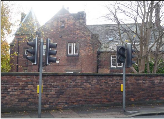
Brick wall at St Thomas Rectory
