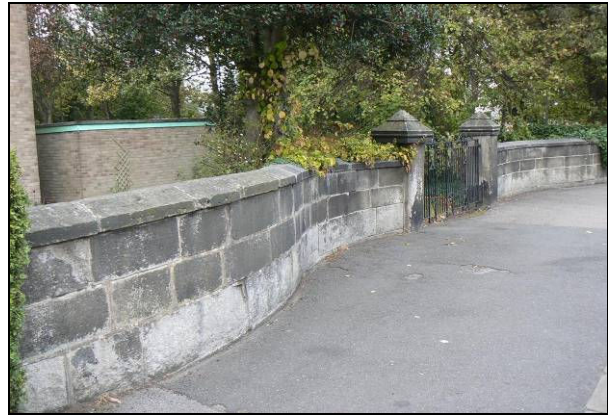
Stone wall in front of Chatsworth Court
