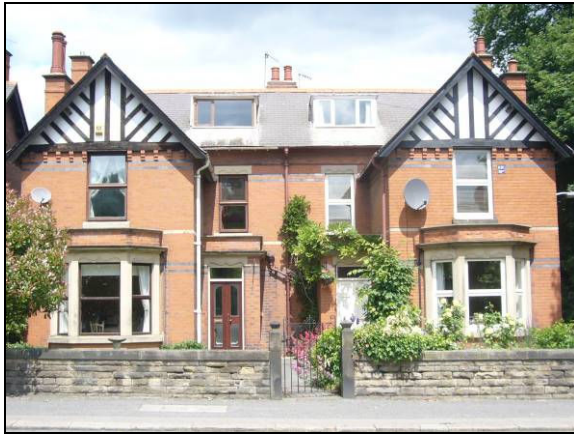
Black & white timber framing gables
