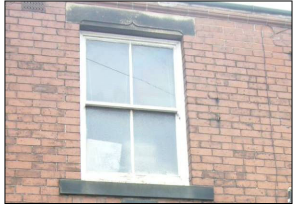
Sash-window with horns
