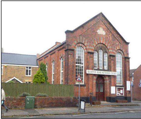
Brampton Moor Methodist Church
