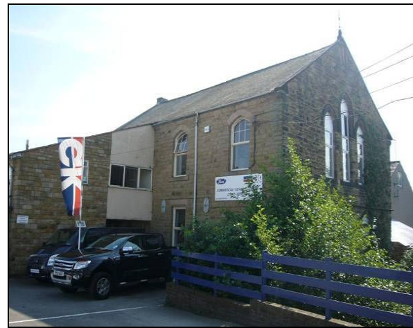
Former Congregational Chapel
