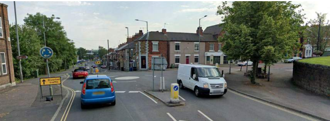
Existing Duke Street Roundabout
