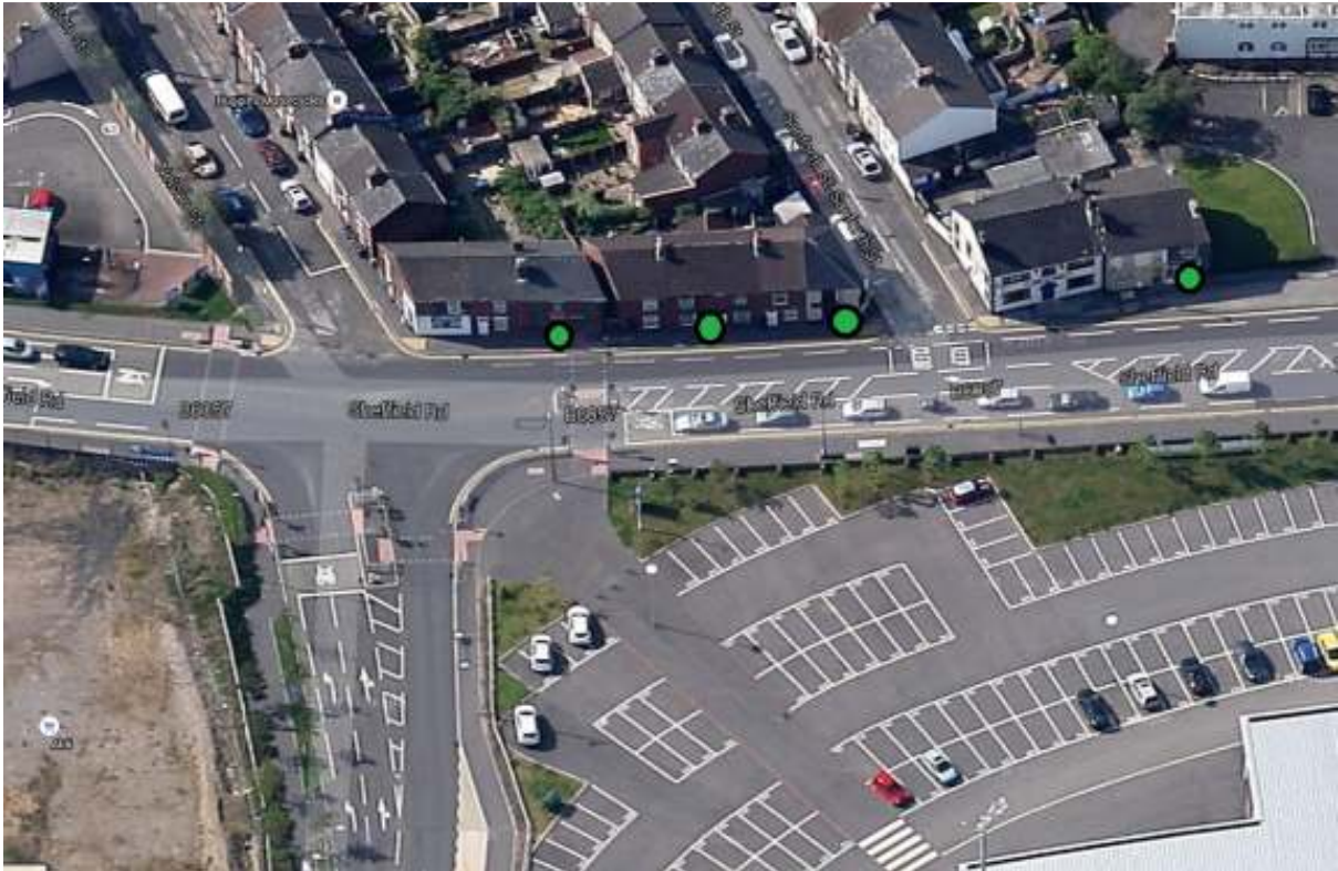
Figure 2: Locations of Diffusion Tube monitoring on the affected façade
