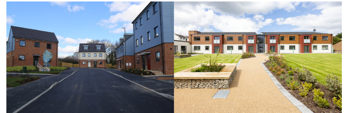
Above left: Badger Croft - Brockwell Court - a new council housing development that has been built on the site of the former Brockwell Court. Each of the new properties has increased levels of insulation.
