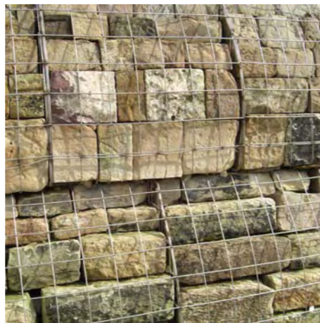
Local Stone Gabion Walls
