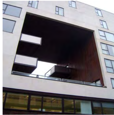
Architectural Window Framing View of
