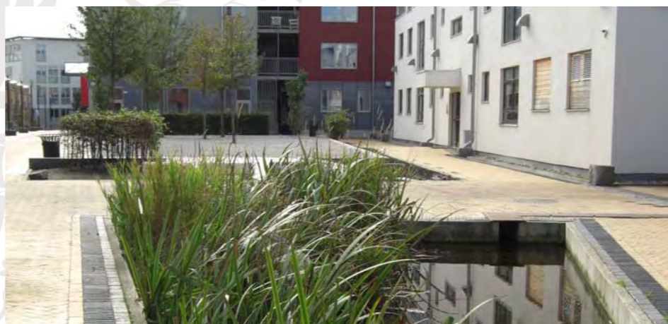
Rainwater Collection in SUDs Systems
