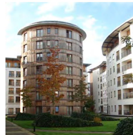
Landmark Residential Tower
