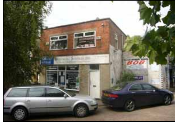
inappropriate extension, High Street
