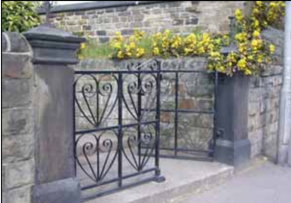
Churchyard gate and gate piers
