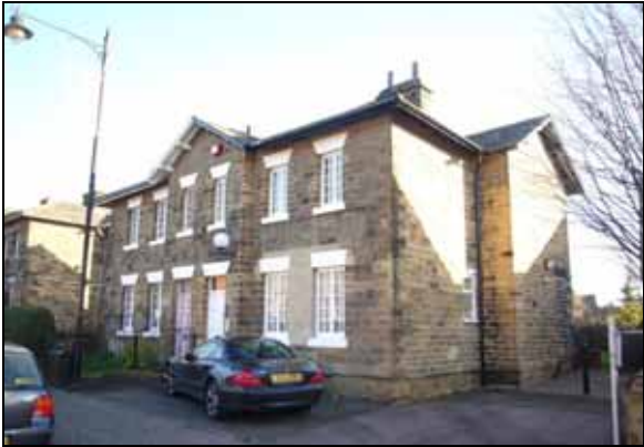
Removal of front gardens for parking
