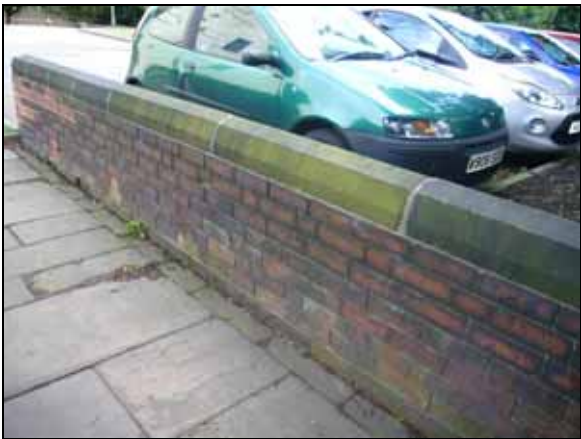
A brick wall with stone coping
