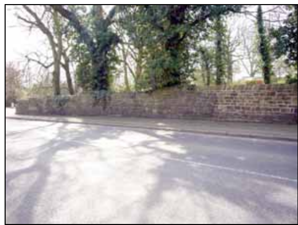
Stone wall along Hall Lane
