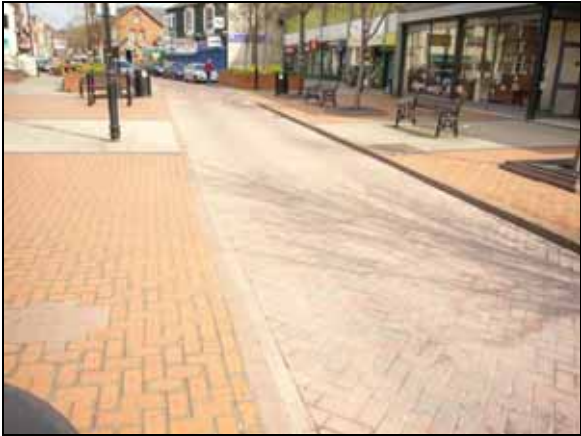
Pattern brick paviers on High Street
