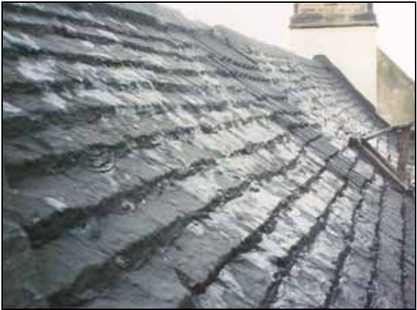
Turnerised stone slate roof (bitumen poured)
