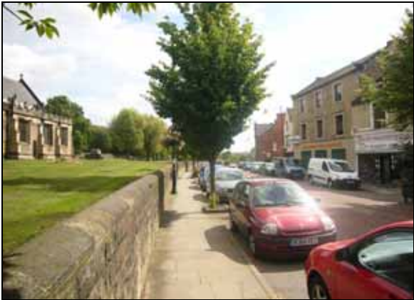
Churchyard retaining wall along Church Street
