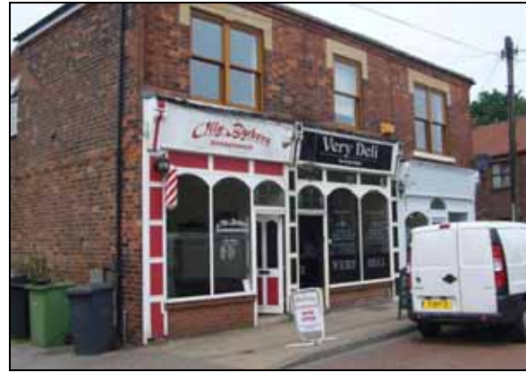
Unsympathetic shop fronts to the building
