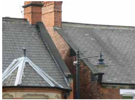
'Welsh' slate roofs
