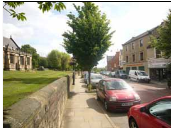
Churchyard retaining wall to Church Street
