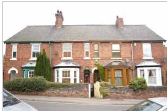
Nos. 27 to 31 Porter Street/1 Rectory Road
