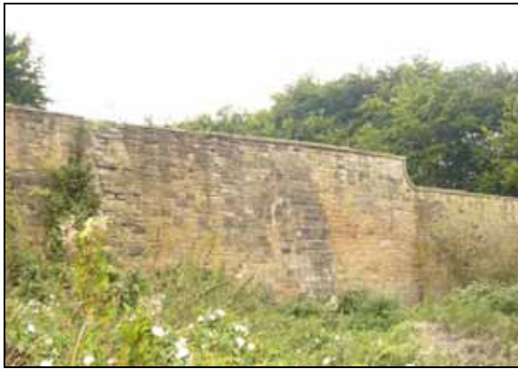
Part of wall at Walled Garden
