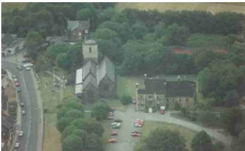
Aerial photo showing Character Area 1
