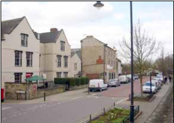
Historic buildings on Church Street
