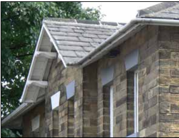
Timber gutters left and UPVc gutters right
