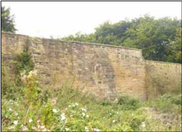
Stone wall along Staveley Hall walled garden
