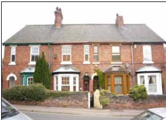
Nos. 27 to 31 Porter Street/1 Rectory Road
