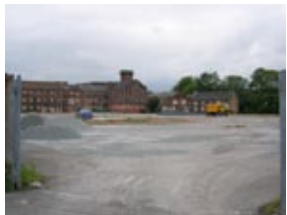
Cleared site of Walton Works
