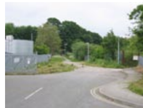
Public route alongside Boythorpe Works
