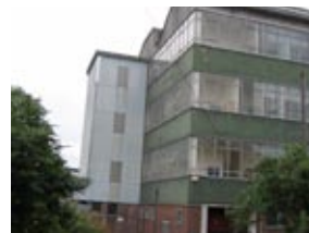
Vacant Wheatbridge Mill building
