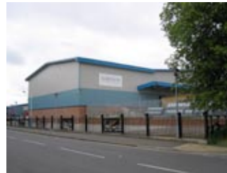
Robinsons on Goyt Side Road
