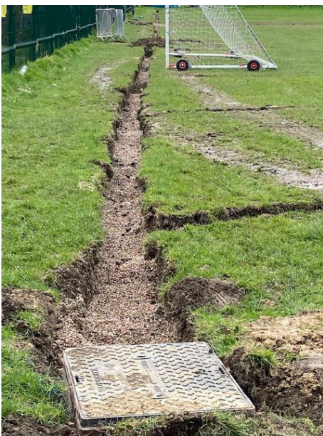
Staveley Miners Welfare Football Club Ltd – Drainage works, now complete
