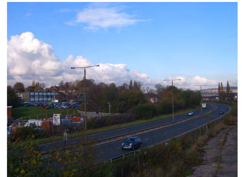
View of A61 from site
