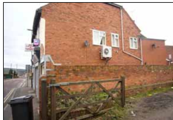
Air condition unit visible from the street
