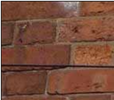
Red Brick wall
