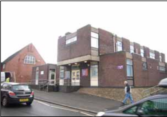
County Council building
