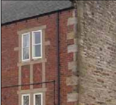
Stone around windows
