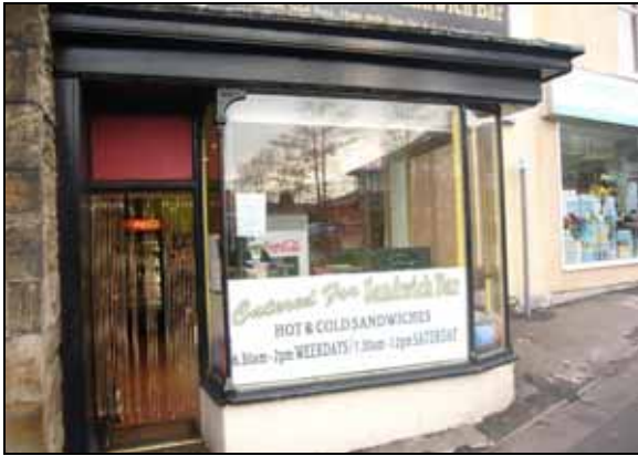
Traditional timber shop front at No. 56
