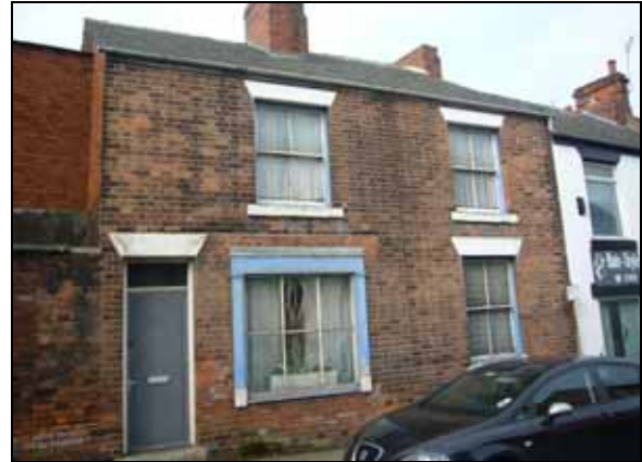
Traditional sash windows at No.23
