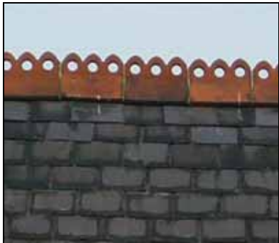
Slate roof with terracotta decorative ridge tiles
