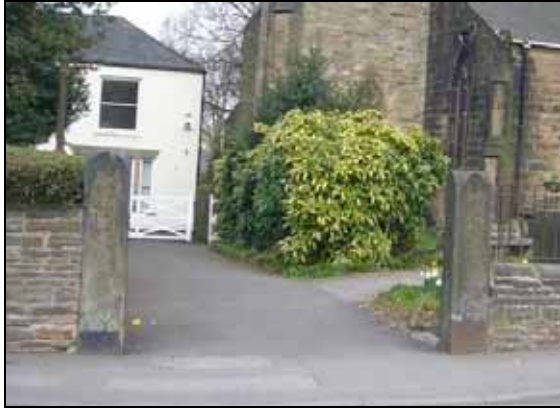
Brick wall with stone copings and railings
