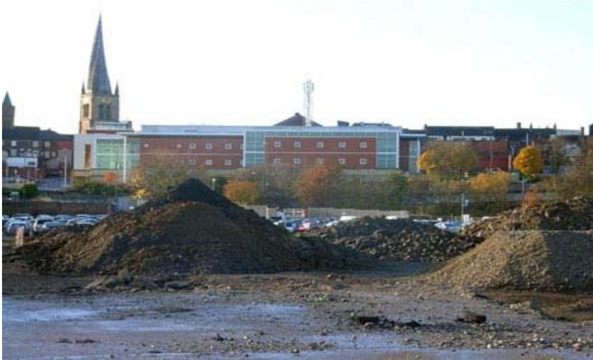
Site for the new canal basin near Chesterfield Town Centre.
