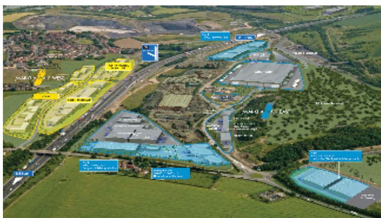
Figure 3.4 Projected Layout of the Completed Markham Vale Development, viewed from the South
