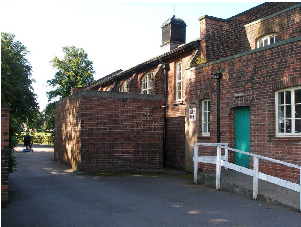
Side elevation showing ramped access to the rear and the brick built air raid shelter which interrupts the rhythm of the Village Hall facade
