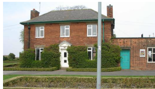
Fig 2.2.12 The caretaker’s house and adjacent refreshment room
