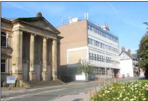
The Telephone Exchange building
