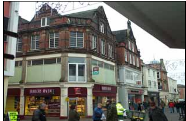
High Street (south side)
