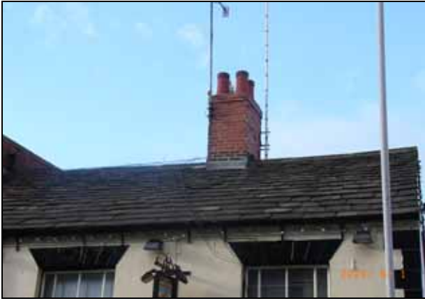
Stone slate roof
