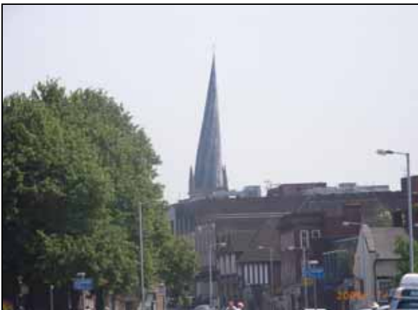
View of the crooked spire and the Market Hall tower from Town Hall
