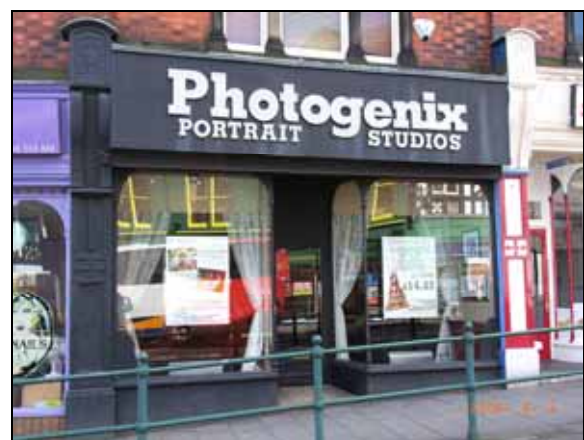
Shop front retaining its original detailing spoilt by contemporary signage
