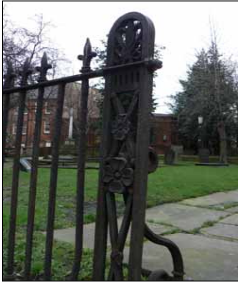
Railings at the Prish Church
