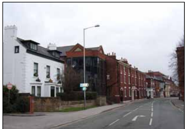
Approach from north-west along Saltergate
