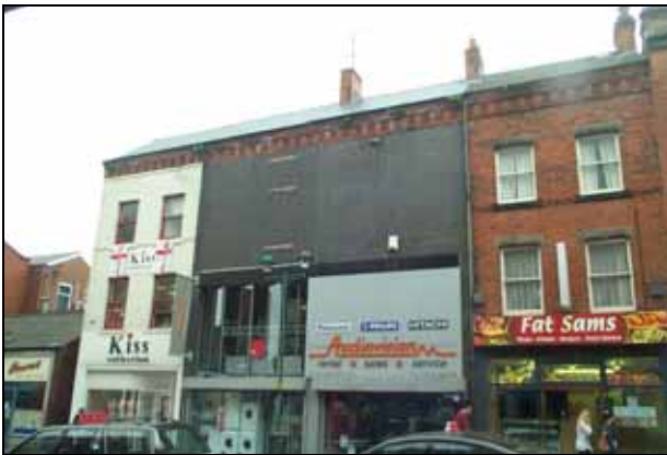
Inappropriate altered building disfiguring the rhythm of the street frontage
