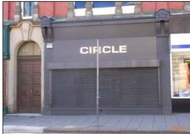
A solid roller shutter with a bulky external housing
