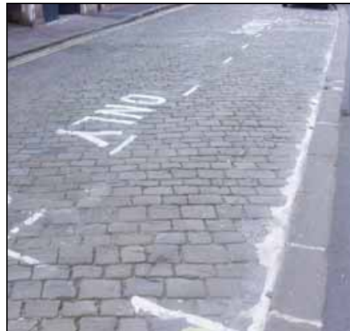
Stone setts and kerb stones, Glumangate
