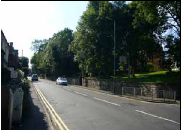
View from north along Sheffield Road
