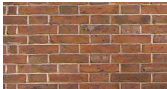
Red Brick wall in Flemish bond
