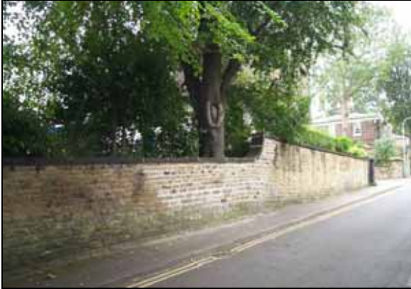
Listed wall to Hurst House
