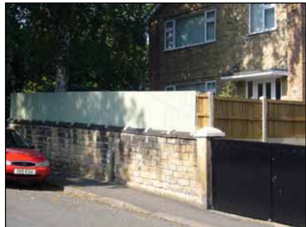
Timber panel fencing on top of stone wall
