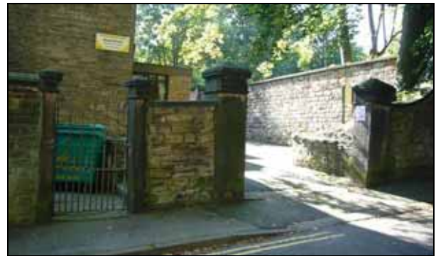
Gate and gate piers
