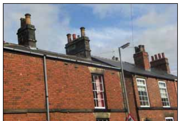
Replacement plastic gutters - right
