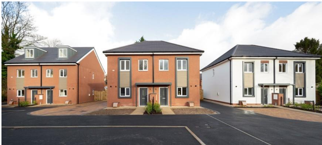
Modular Construction properties at Heaton Court, Chesterfield
